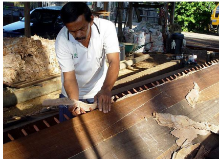
Craftsman applying the caulking bark
