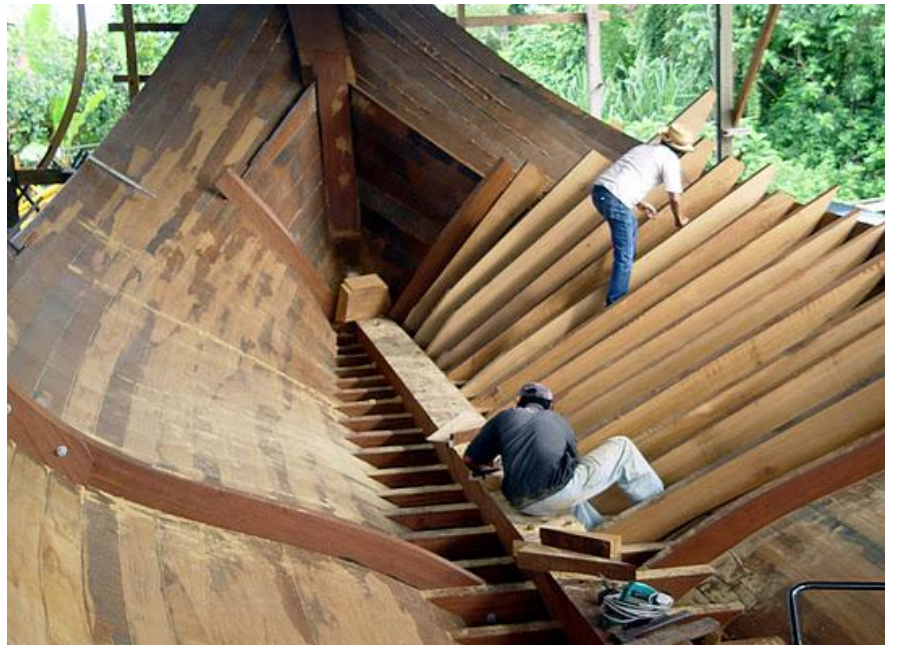
Frames are fitted
