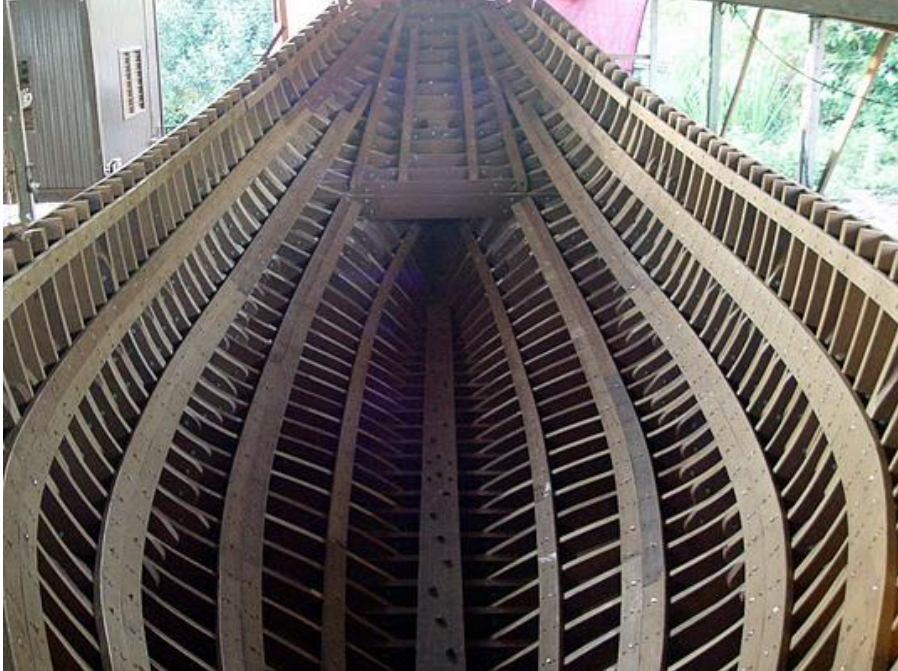
Frames and stringers are in place
